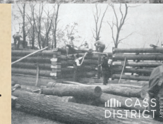
Building the Pioneer Log Cabin, Cassopolis, May 23, 1923. Cass District Library Collections.
