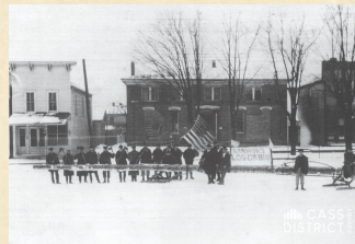
1860 Cass County records building, taken during the winter of 1922-1923 when it was used as the Masonic Temple. Men in front were transporting a log to the site of the Pioneer Log Cabin to be built during the upcoming spring. Cass District Library Collections.
